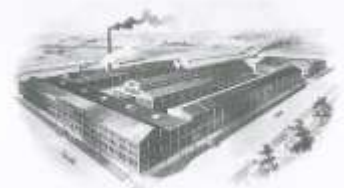
Naale Enaine & Boiler Works
