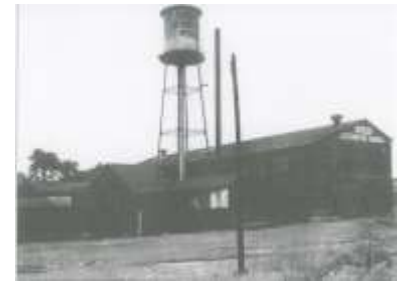
Heisler Locomotive Works
