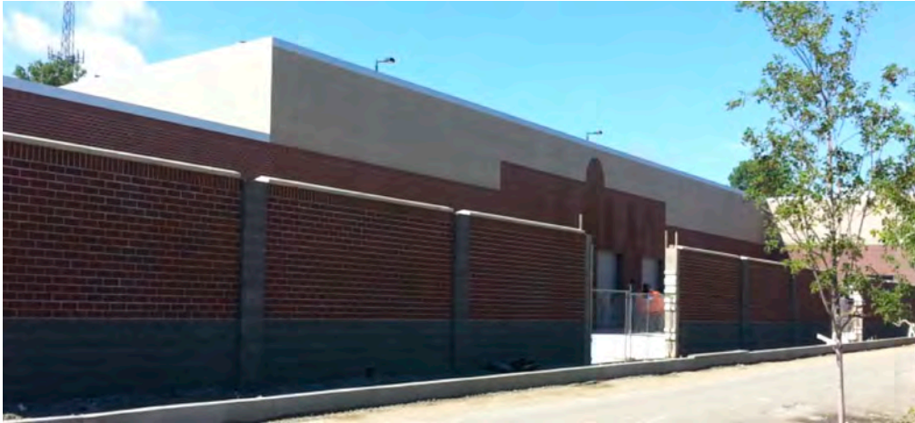
New EMTA Lift Facility on 14th Street
