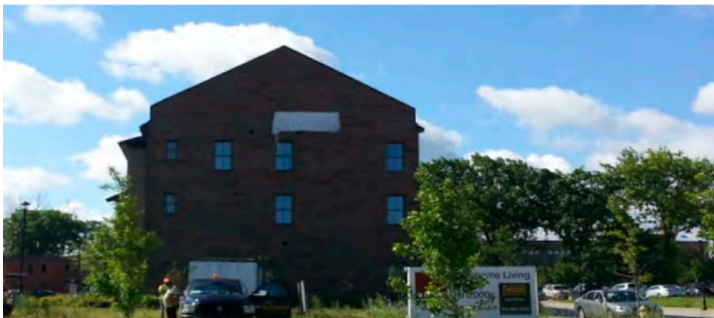
Commercial space at Union Square on 12th Street
